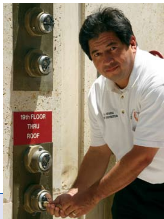
Gerald Esparza, Fire Inspector, installing FDC plug.
