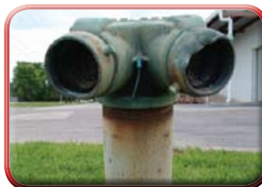
How would you connect to this FDC in an emergency?
