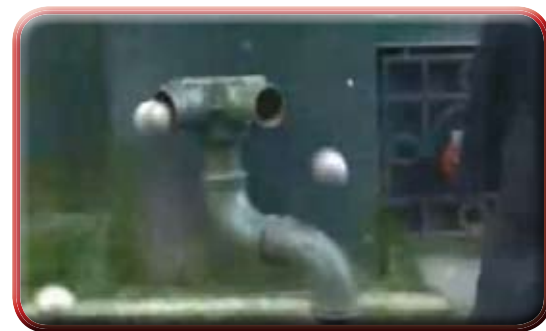
Open FDCs are so common that they've become creative props for television advertisers. This scene showing baseballs popping out of a siamese connection was aired twice during this year's Super Bowl.
