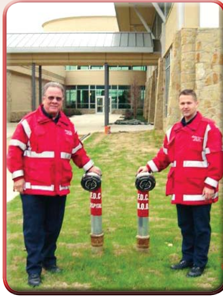
Fire Marshal David Barnes and Fire Inspector John Ard showing off installed StorzGuard caps.
